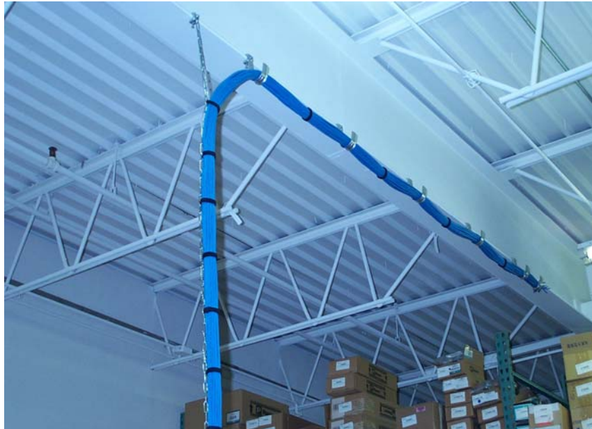
Figure 7-5: Example of Cable Vertical Transition with Chain Support.
